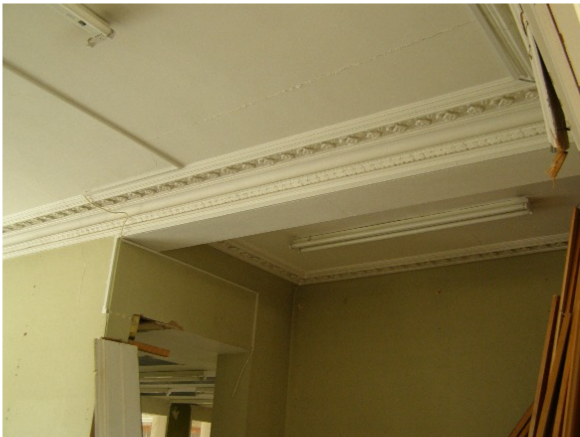
Figures 20 a & b. Rear section of main room suite on ground floor showing simplified cornice in small 1906 extension.
