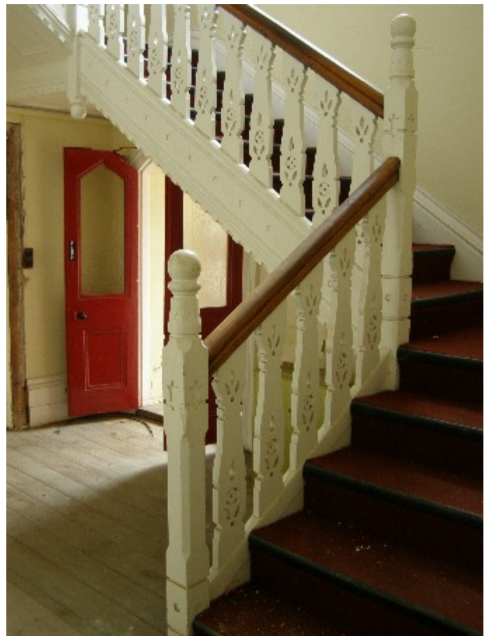
Figures 33 a & b. Lower section of main staircase, with internal front door shown closed and open. Note the foliate motif used in the balusters.
