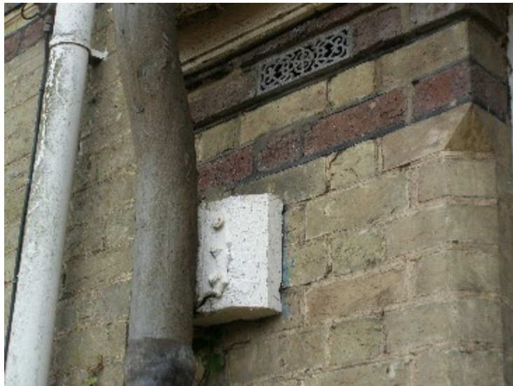
Figure 59. Detail of fixing on lead soil pipe in Figure 58.
