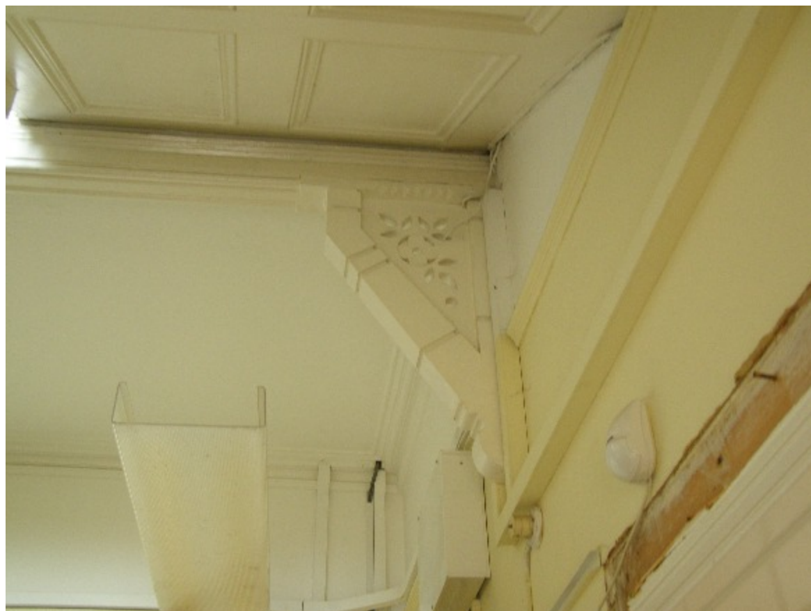
Figure 39. Detail of bracket where uppermost section of staircase meets the landing.
