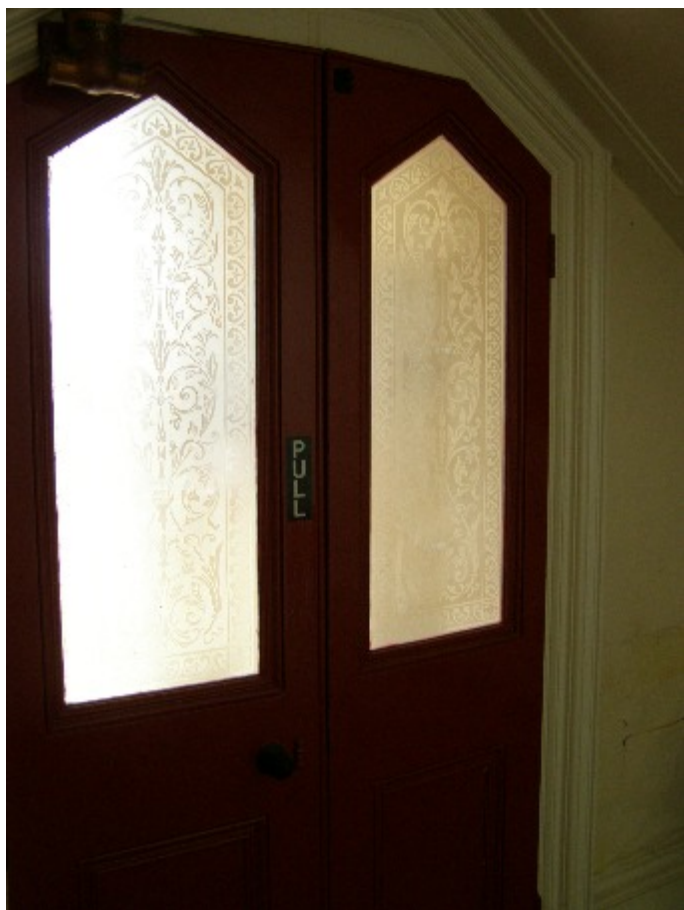
Figure 49. Detail of interior of inner front door, showing etched glazing.
