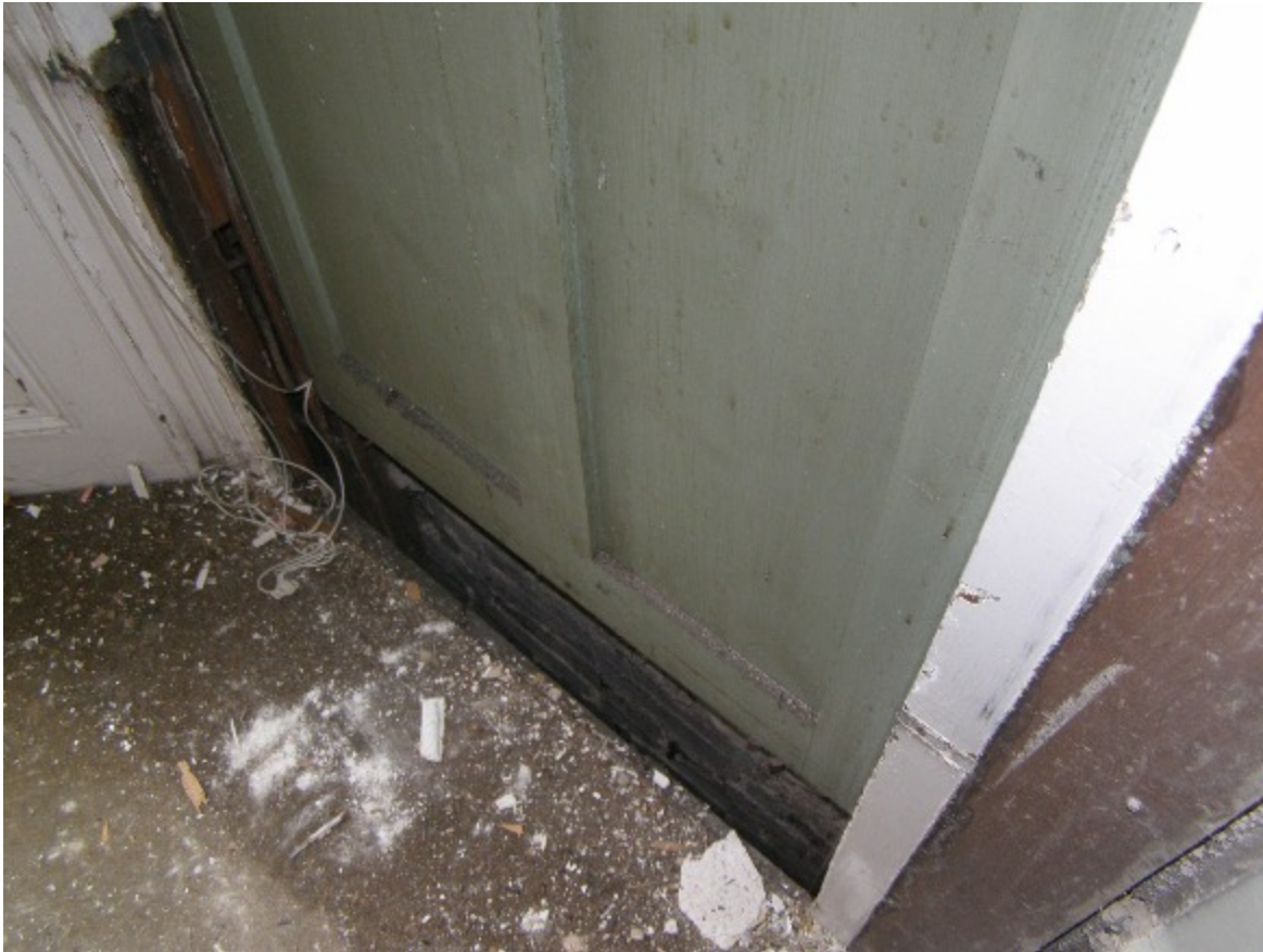
Figure 23. Rear section of main room suite on ground floor, interior of main bay, showing the recess partly below ground in which the shutter is normally stored.
