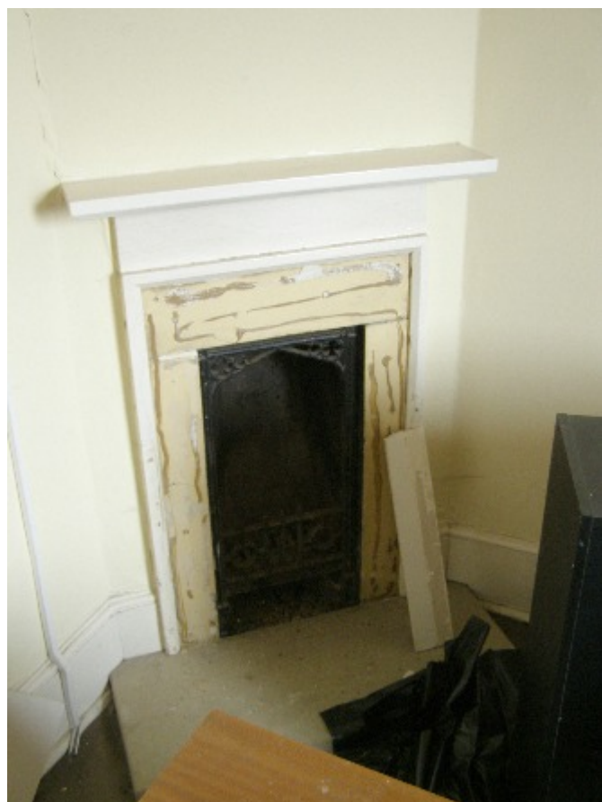
Figure 47. A fire place on an upper floor, with a plain surround and cast iron grate.
