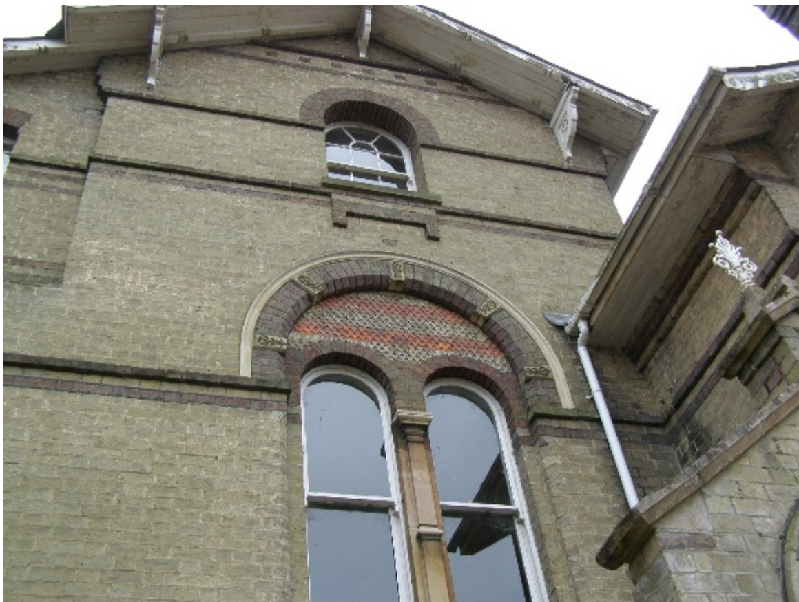
Figure 7. Staircase window in detail, principal elevation, showing saltire mouldings in brick of tympanum, and deep, bracketed verges to gable.
