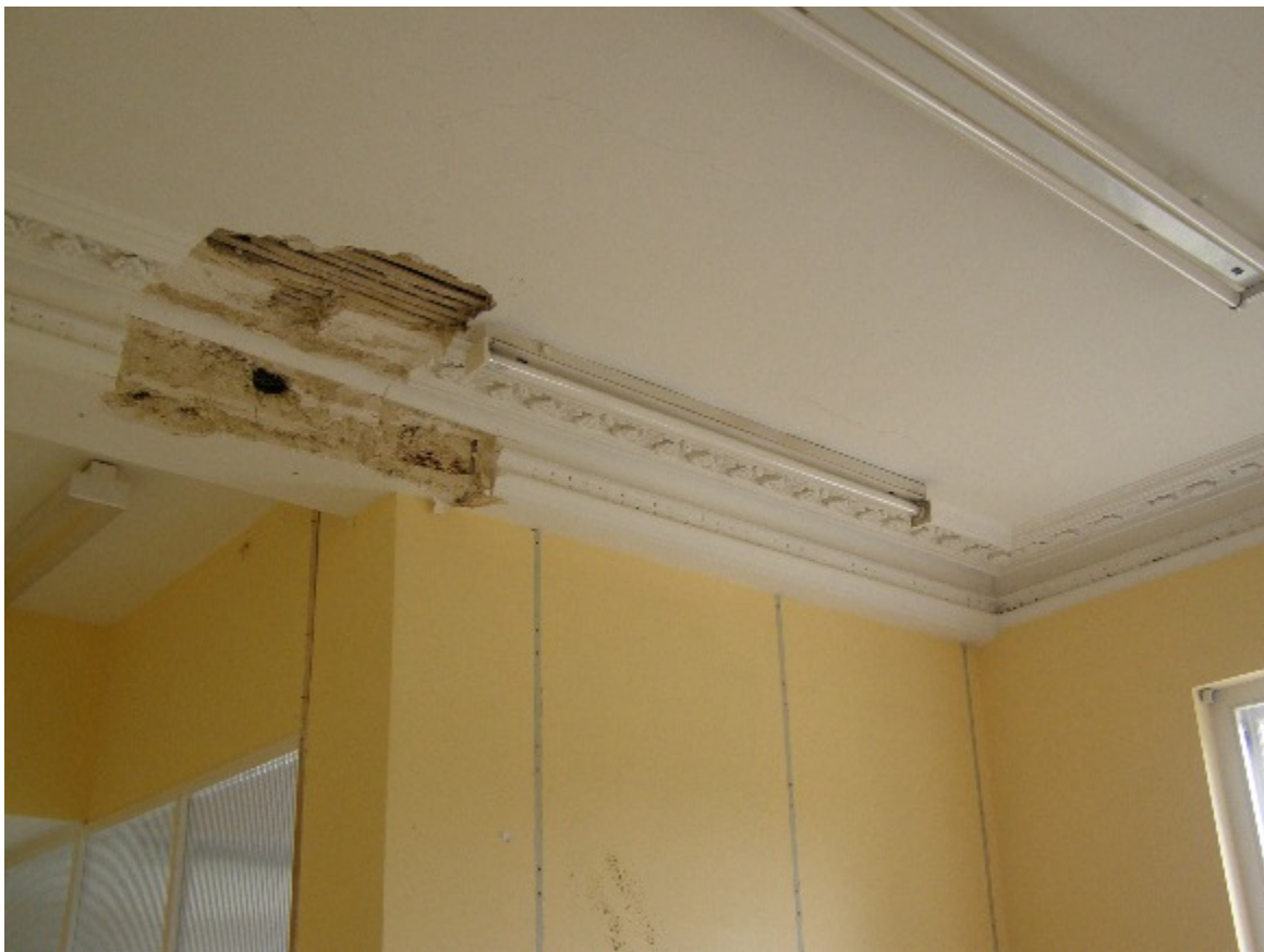
Figure 17. Front section of main room suite on ground floor showing cornice from which a portion had previously been removed.
