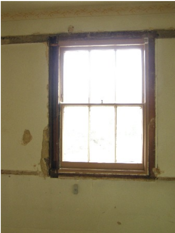
Figure 24. Interior of “3 over 3” sash window on front ground floor in the service area of the house.
