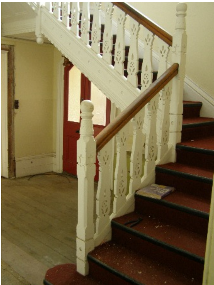
Figures 33 a & b. Lower section of main staircase, with internal front door shown closed and open. Note the foliate motif used in the balusters.
