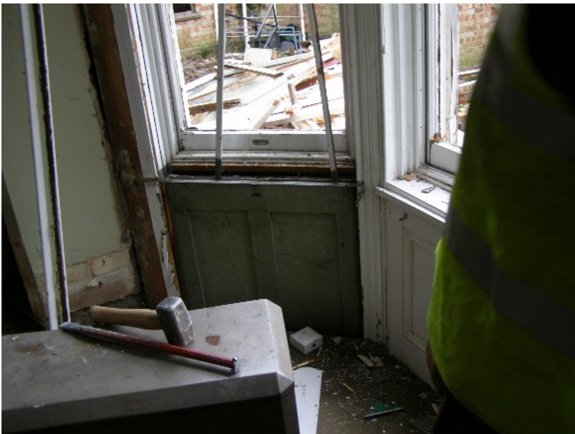
Figure 22. Rear section of main room suite on ground floor, interior of main bay. Detail of lift up shutter.
