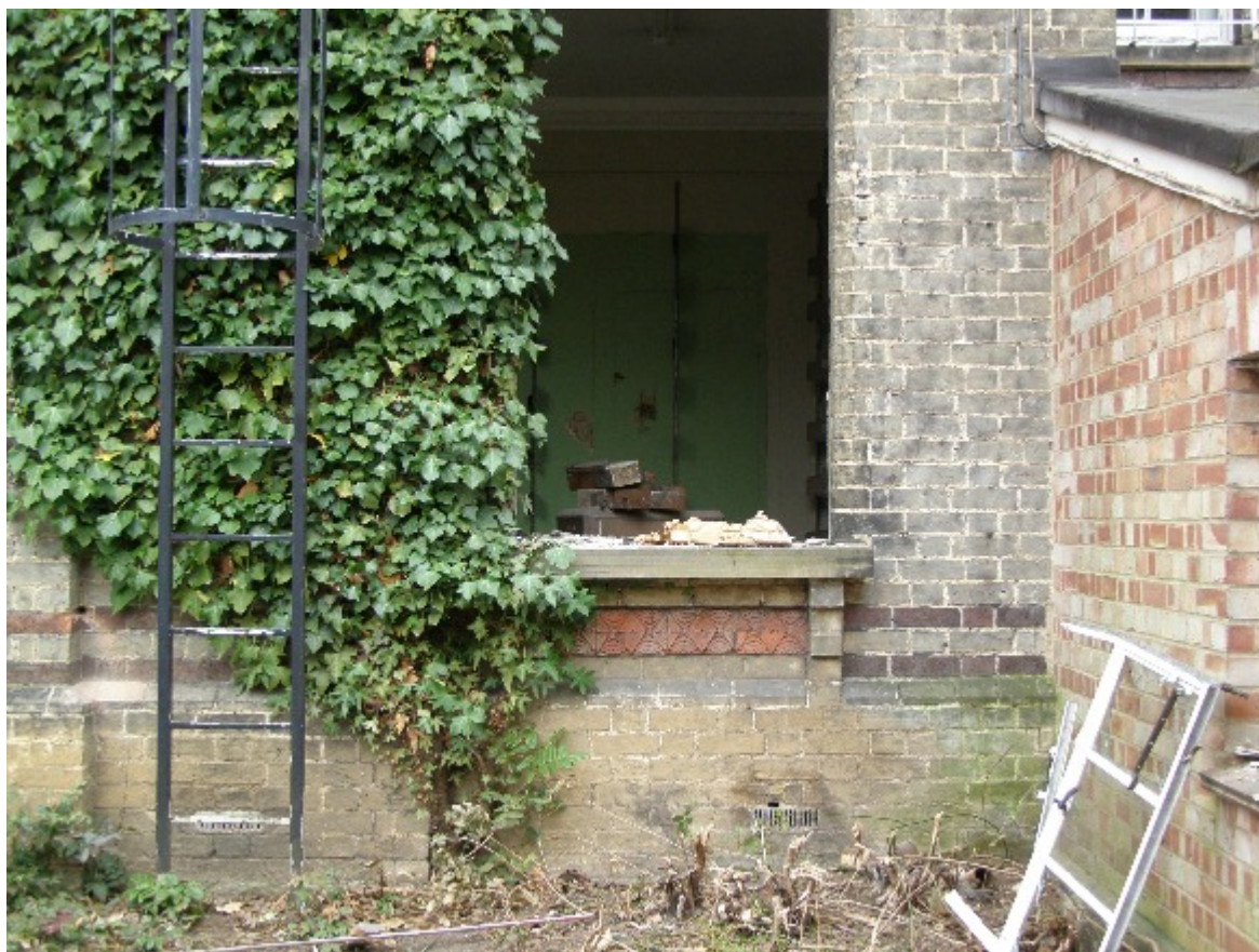
Figure 54. Window opening on rear elevation with ornamented bricks below sill.
