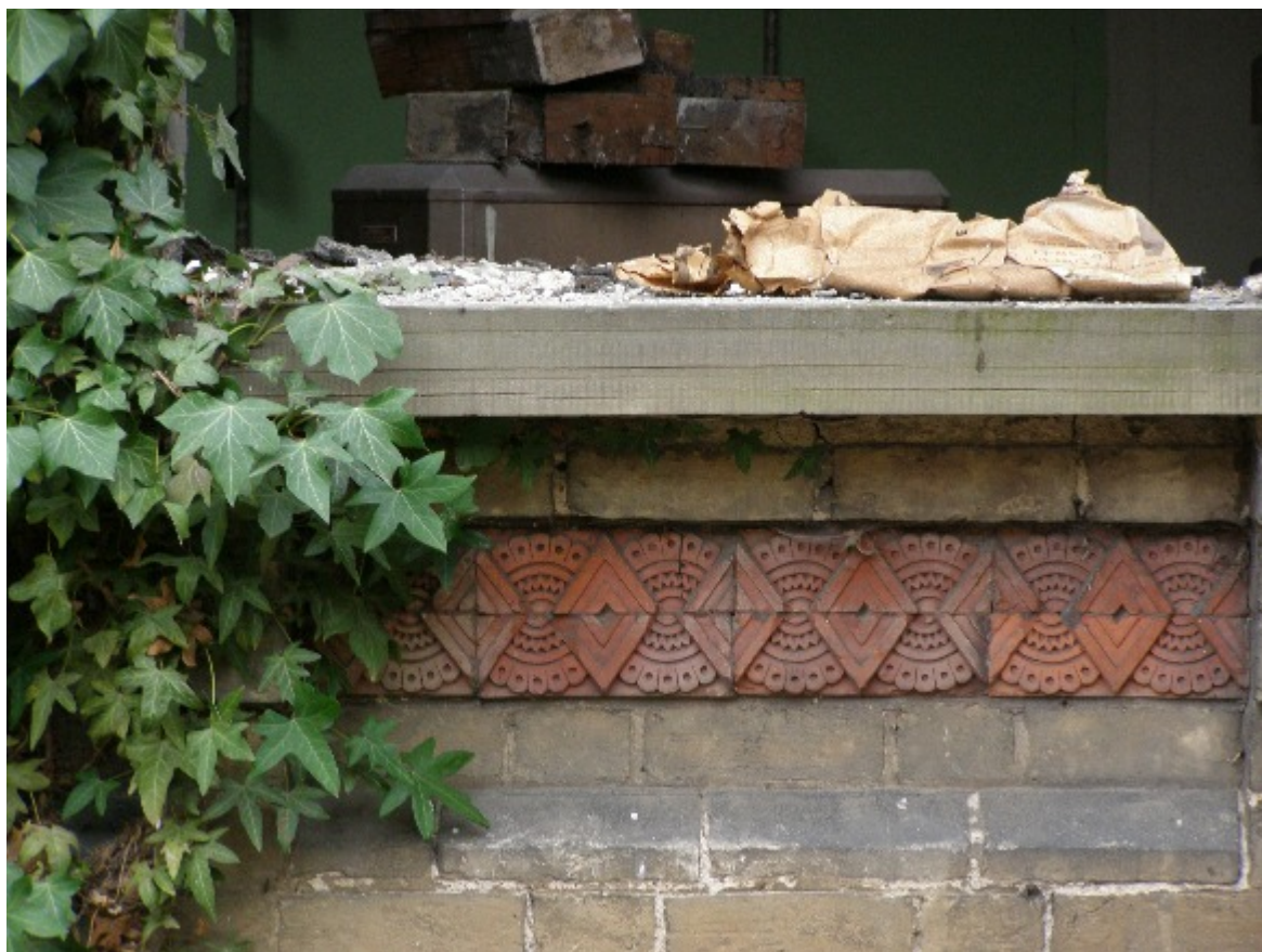
Figure 55. Detail of ornamented bricks below sill on window opening in Figure 54. This motif was not seen elsewhere on the building.
