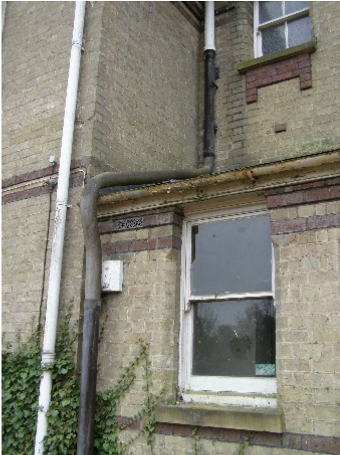
Figure 58. Lead soil pipe on east elevation.
