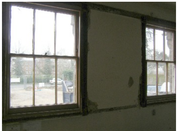
Figure 25. Interior of further “3 over 3” sash windows on front ground floor in the service area of the house. (Photograph enhanced to improve exposure.)
