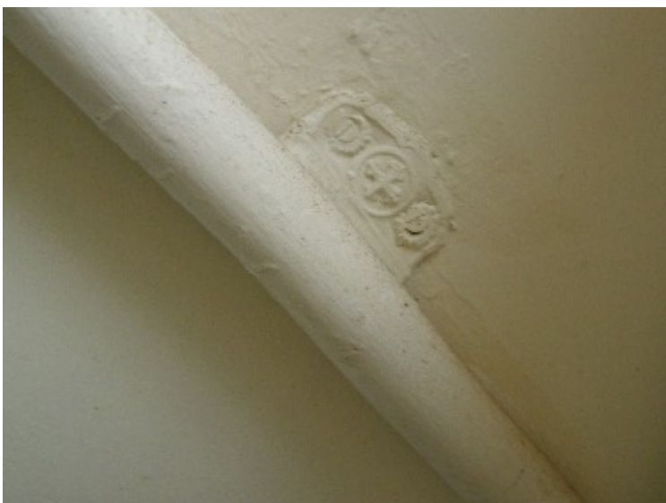
Figure 60. Detail of fixing on flush pipe in ground floor WC.
