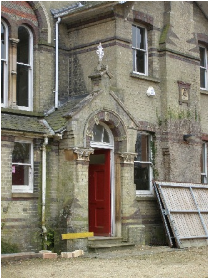
Figure 7. Staircase window in detail, principal elevation, showing saltire mouldings in brick of tympanum, and deep, bracketed verges to gable.
