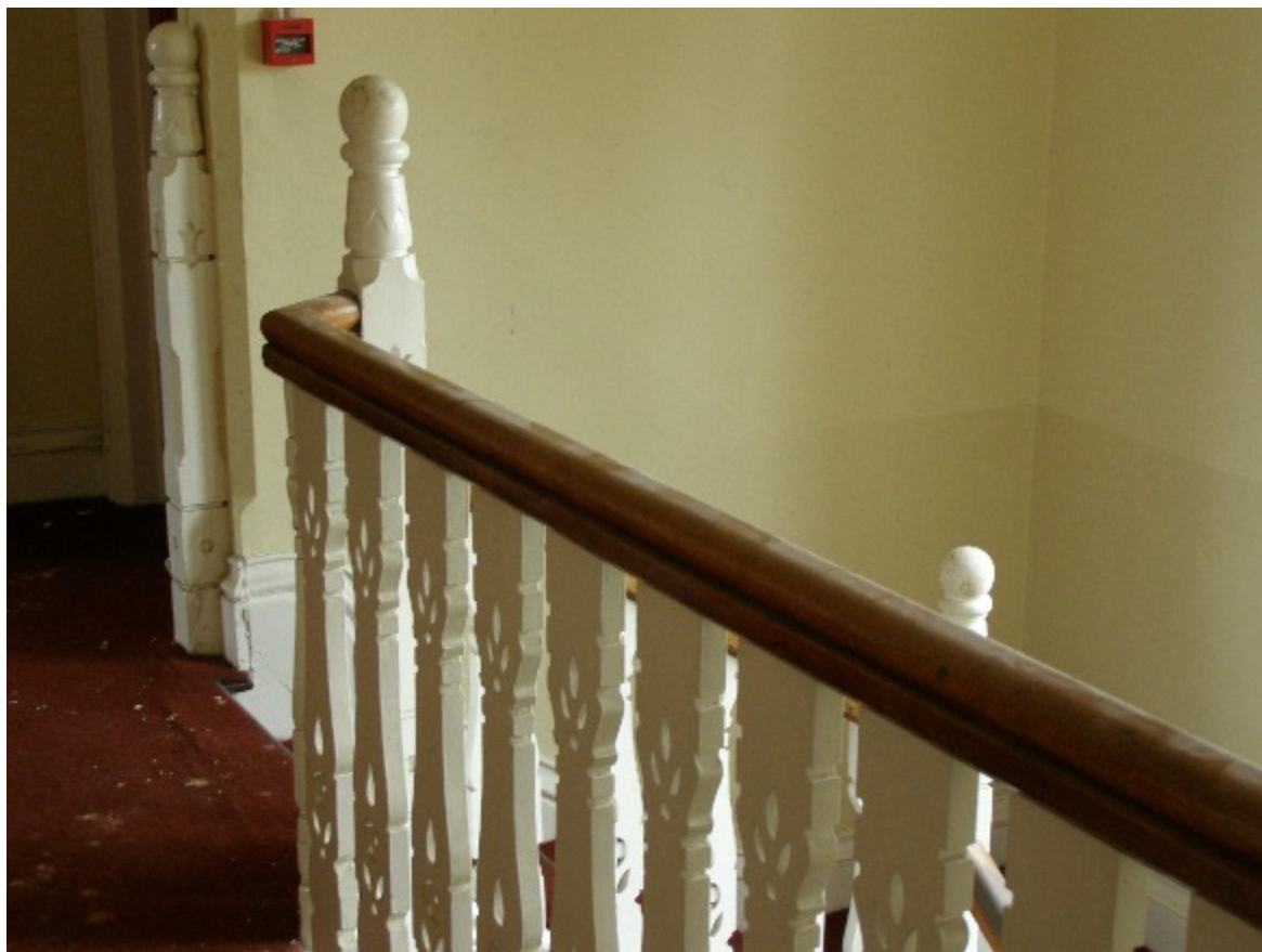
Figure 38. Detail of landing balustrade seen from landing, showing newel posts.
